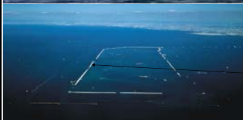
Sea wall Construction
